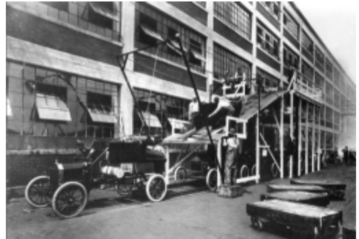
1913 Ford production line. Picture by Ford
