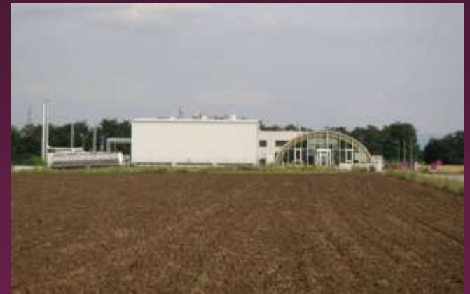
A biodiesel refinery In Germany
