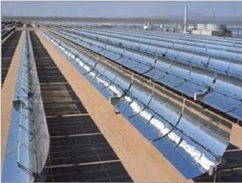
Solar-thermal array. Picture by US Dept of Energy, Public Domain
