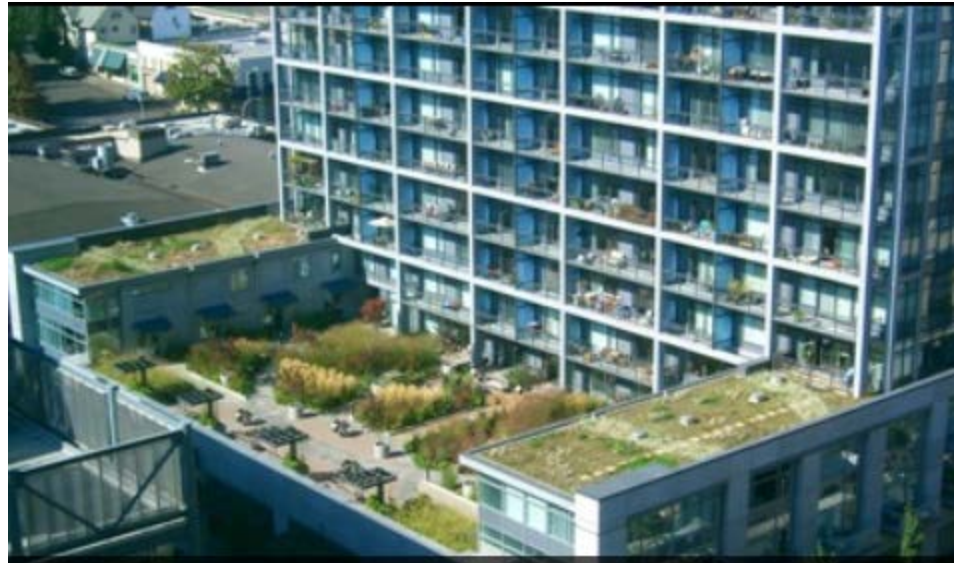
Louisa Apartments, Portland. Picture from portlandonline.com
