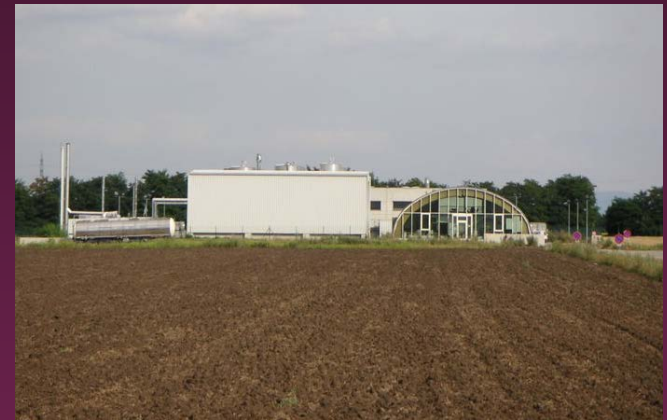
A biodiesel refinery In Germany
