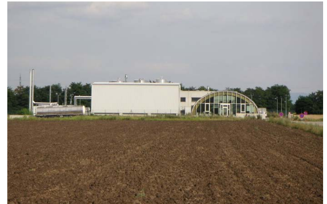
A biodiesel refinery In Germany
