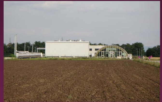
A biodiesel refinery In Germany
